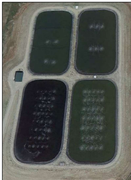
Figure 1: Multiple pond aerated lagoon system, above. Google Earth
