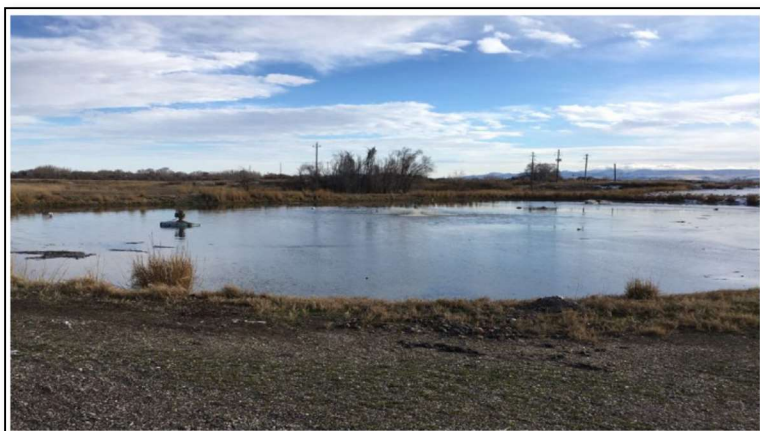
Figure 10: One of three aerated ponds at a 0.3 MGD municipal lagoon system. Photo courtesy of Mark Sembach
