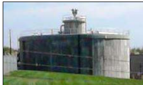
Figure 18: A side benefit of treating the collection system with PBII, was the quantity of solids that needed to be removed from the anaerobic digester decreased.
