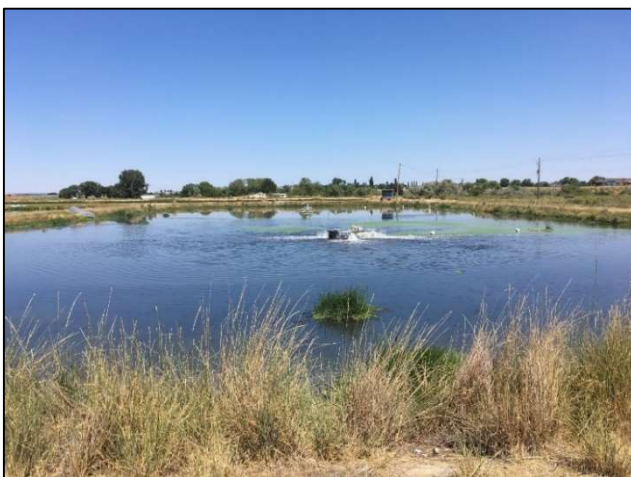
Figure 2: A surface aerator on an aerated lagoon. Photo courtesy of Mark Sembach.
