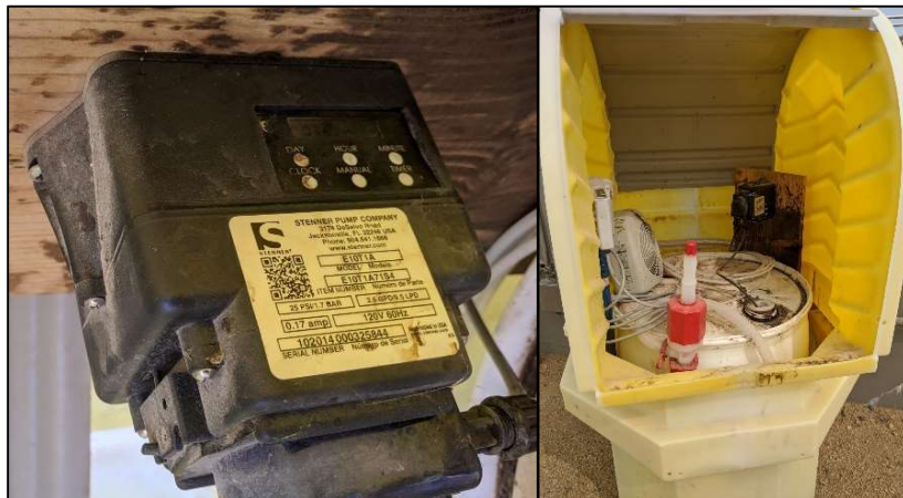
Figure 10: The Candy Carbon feed system consists of a programmable peristaltic metering pump and the reservoir for the product. Photos courtesy of Marshall Davis
