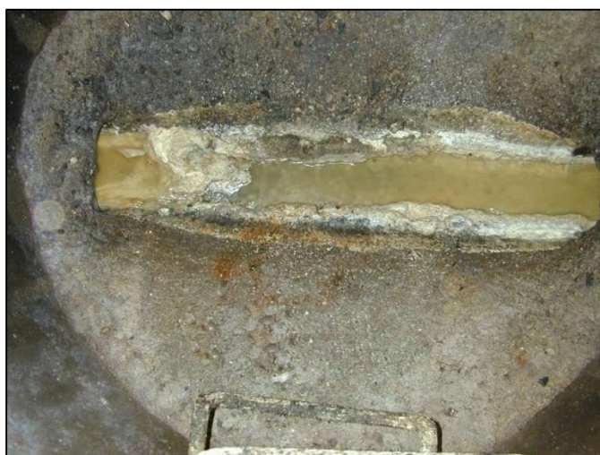
Figure 2: Looking down into a manhole one can see significant buildup of FOG on the lateral line from a commercial establishment. The lateral connects the business to the sewer system. One can also observe corrosion to the concrete as well as the metal steps (bottom of photo).
