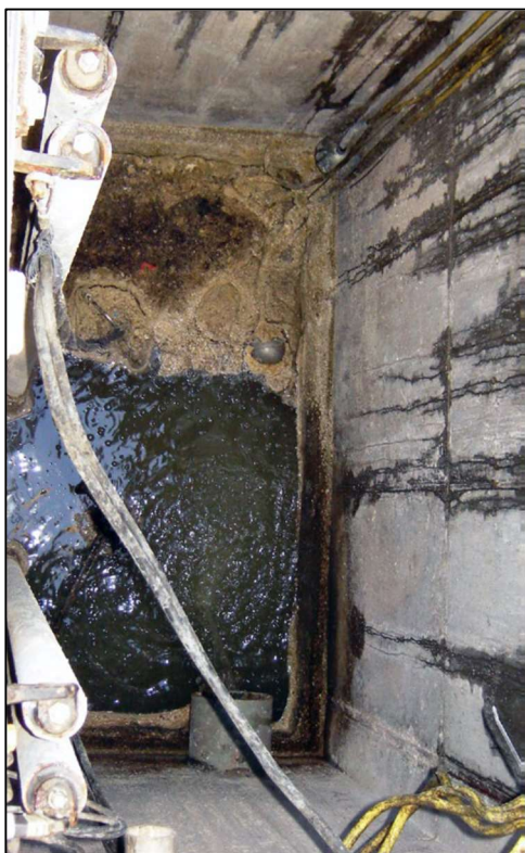
Figure 17: The lift station prior to treatment with PBII. FOG and precursors were dark colored and difficult to remove. Degreasers being used had only limited effectiveness. Photo courtesy Mark Sembach, BioLynceus.
