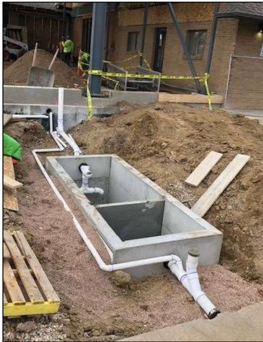
Figure 4: A new grease interceptor (GI) being installed at a restaurant. A multiple chamber design with a baffle(s) between the chambers is common. The design is such that FOG floats to the surface in the first chamber while the liquid phase goes under the baffle wall. Remaining FOG then floats to the surface of the second chamber. There is typically a baffle or other arrangement to prevent the floating FOG to leave the second chamber. The liquid phase will be drawn from the bottom.
