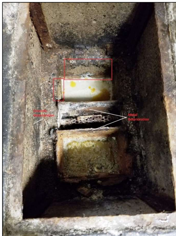
Figure 5: Grease interceptor (GI) exhibiting significant damage due to the corrosive nature of FOG. Top center one can see exposed soil where the concrete is missing. One can also observe extensive damage to the concrete parts of the structure to the left of the picture. In the middle of the photo observe the lines indicating areas of significant corrosion to exposed metallic parts.
