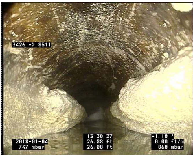
Figure 8: The image of the substances as they go down the drain is significantly different from what is observed in the sewer. One sees large masses of deposits that appear to be more “soapy” than oily or greasy.
