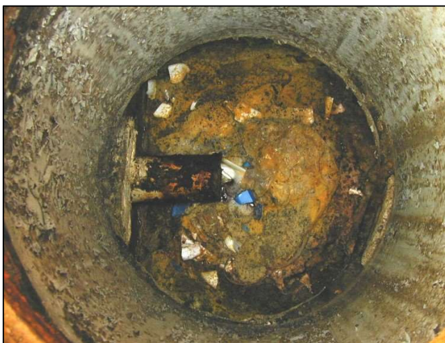
Figure 11: Most commercial establishments that discharge FOG are required to install and maintain a 'grease trap' or grease interceptor (GI). One can see here a poorly maintained GI containing not only FOG but also waste such as plastic and paper cups and other debris that has no place in a sanitary sewer system.
