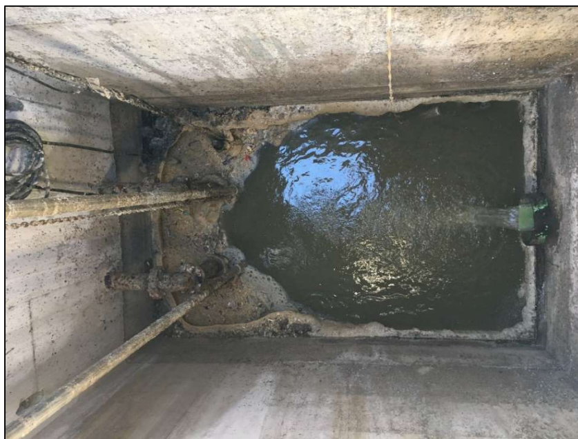
Figure 21: The lift station before starting treatment with PBPP. Notice the FOG coating the walls and 'climbing' the piping and chains. Photo courtesy Herb Fancher, BioLynceus.
