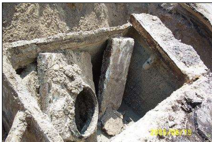
Figure 6: Grease interceptor completely collapsed due to corrosive effects of FOG.
