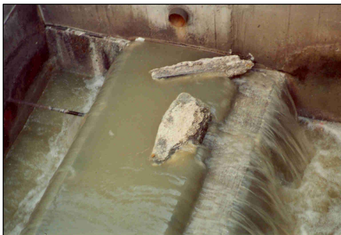
Figure 1: Floating pieces of FOG at the effluent of the grit chamber of a wastewater treatment plant. 1
