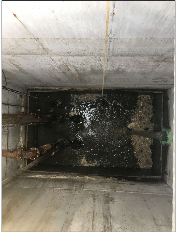
Figure 22: After 3 months of treatment with PBPP the lift station equipment structure and equipment were virtually free of FOG buildup as can be clearly seen in the photograph. Photo courtesy Herb Fancher, BioLynceus.
