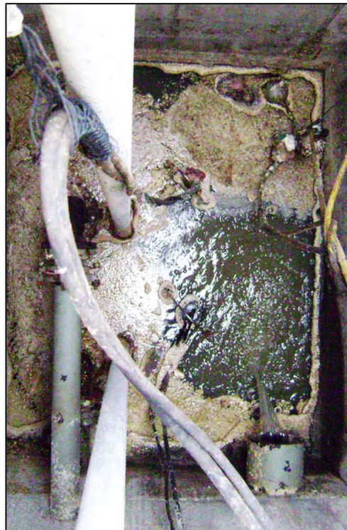
Figure 18: The city's lift station one month after beginning treatment with PBII. There were fewer solids in the lift station. Solids were now lighter in color and softer in texture so were easier to remove. Photo courtesy Mark Sembach, BioLynceus.
