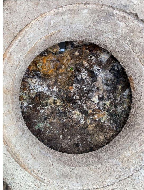
Figure 15: A view into this manhole exhibits a substantial amount of FOG that will soon create more serious problems and costly resolution. Bioaugmentation applied now can save significant money and effort down the road. Bioaugmentation is the preventative maintenance alternative to brute force. Photo courtesy Kathy Kelly. BioLynceus.
