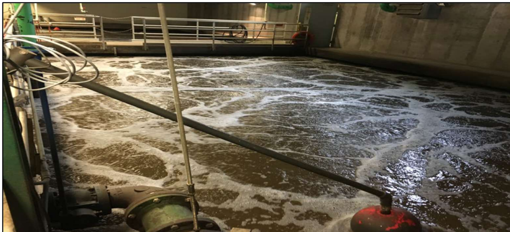
Figure 6: Aeration basin after treatment with PBII with normal foam.
